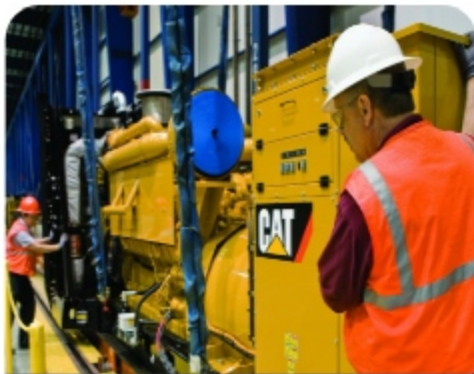
Diesel Generator Installation
